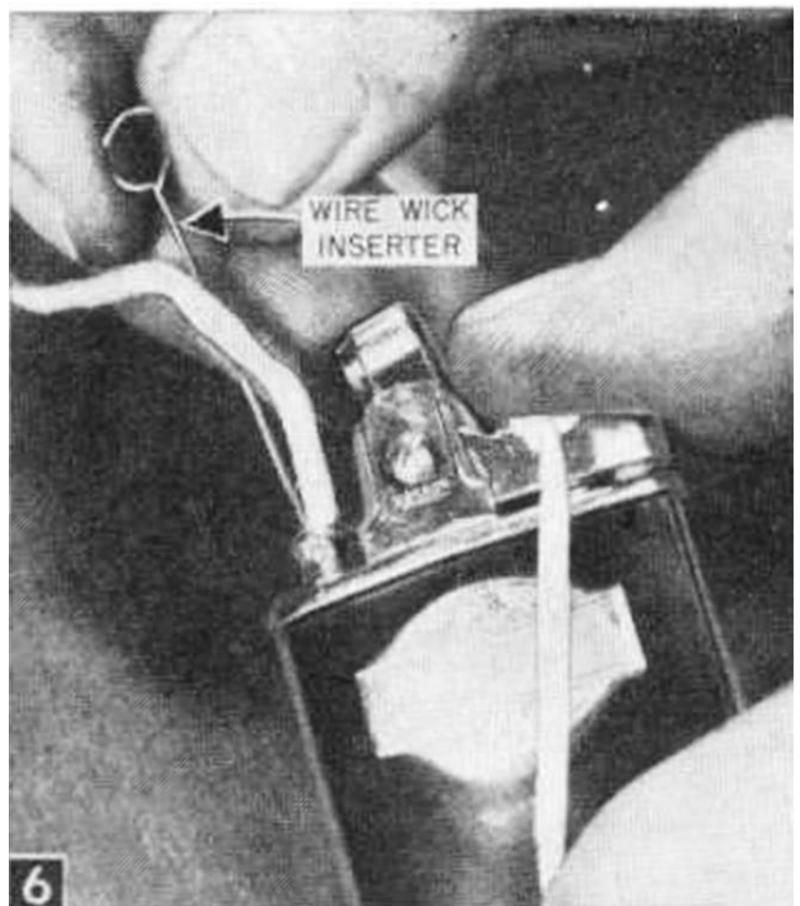
Push all but about 1 in. of wick into lighter, using a short piece of stiff wire. Reach into fuel chamber opening with tweezers, wire or crochet noodle to grasp other end of wick and pull it out.
