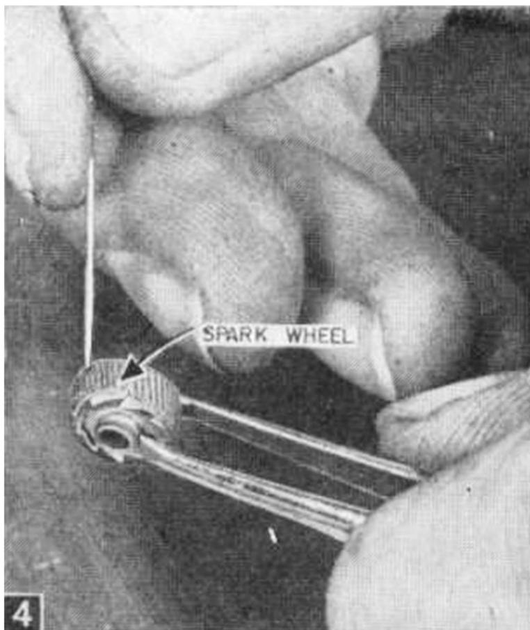
With a large needle or very sharp awl, remove grit, dirt and pieces of flint from spaces between serrations of spark wheel; again brush-clean with solvent. Replace wheel if any serrations are worn.
